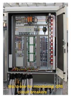
The system is intended for continuous monitoring of the present parameters and predicted calculation of the main technological values of high-voltage SF6 circuit breakers. Also, it is designed to determine and provide information to the duty staff on an occurrence, development and nature of emergency processes.
